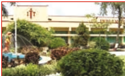
UNIT NO.1 NASIK PLANT
